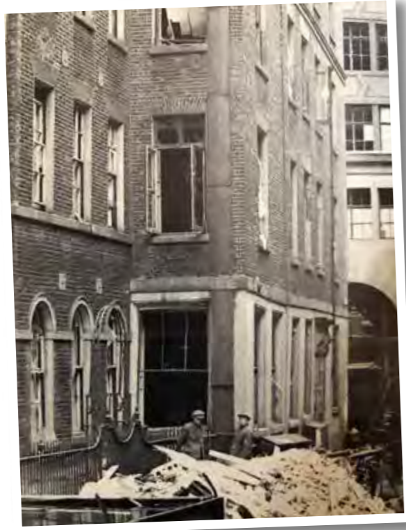
Bomb damage to Frederick's Place, the City home of Price Waterhouse
